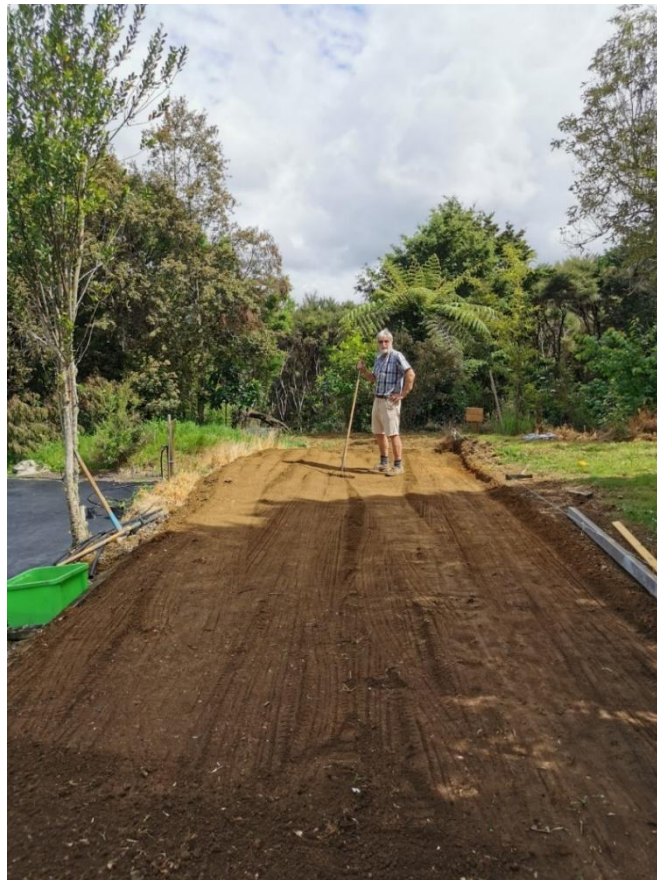
The new hardstanding area. Erik leaning on his tools.
